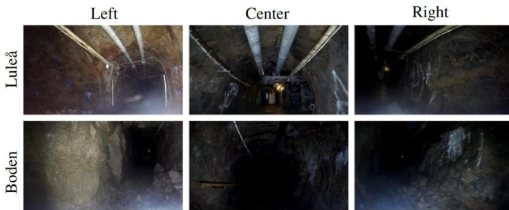
FIGURE 12.24 Photos from an underground tunnels in Sweden.
