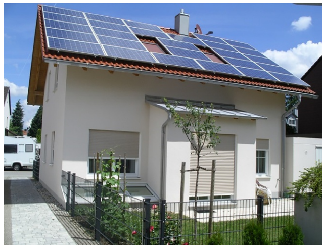
FIG. E12.1.1 High-efficiency, single-family dwelling with PV system and ground-water heat pump. (Courtesy of E. F. Fuchs).
