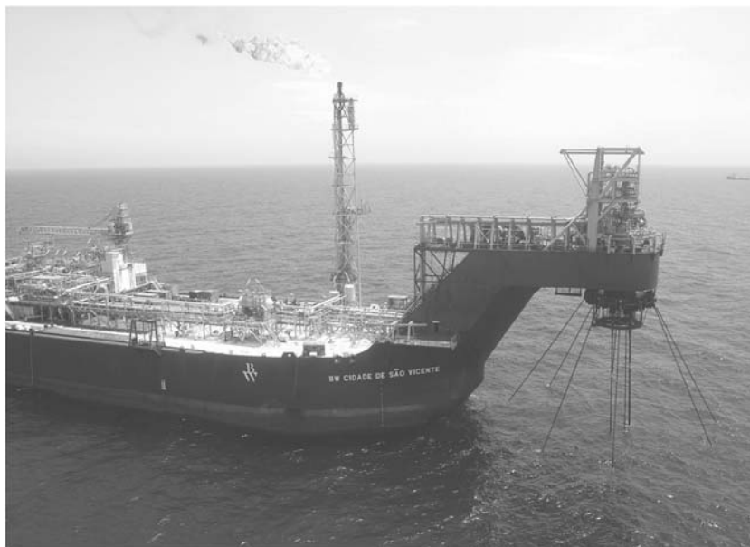
Figure 4.6 Flare (flare stack), designed to make controlled and safe burning of large gas inventories.
