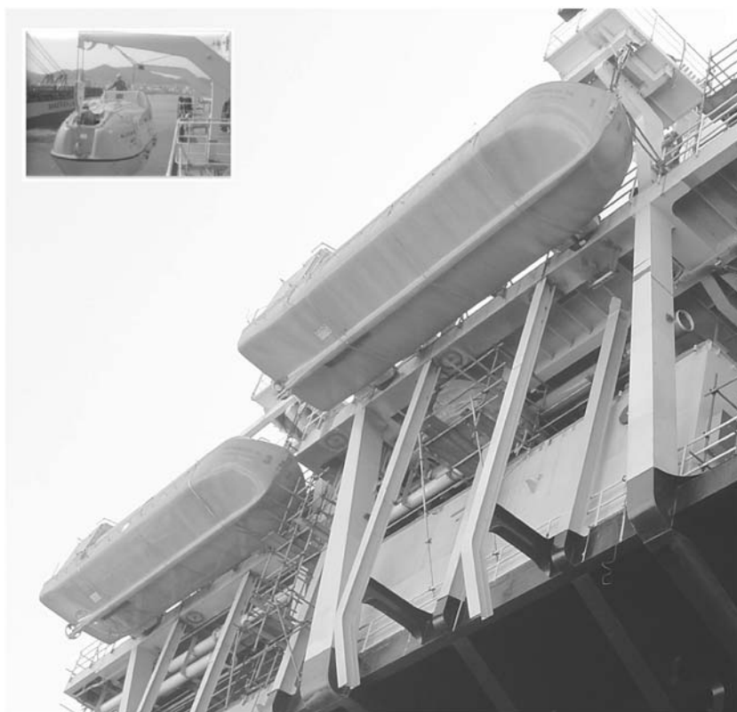
Figure 5.5 Construction and assembly phases of the FPSO rig. Bottom view of a set of two conventional lifeboats supported by the cables of a fixed davit in the launching position. The lifeboat keels are always positioned directly over the sea, with no need for the rotational movement of the davit during launch. The detail view shows the view from the deck of another fixed davit. FPSO , Floating production, storage, and offloading system.
