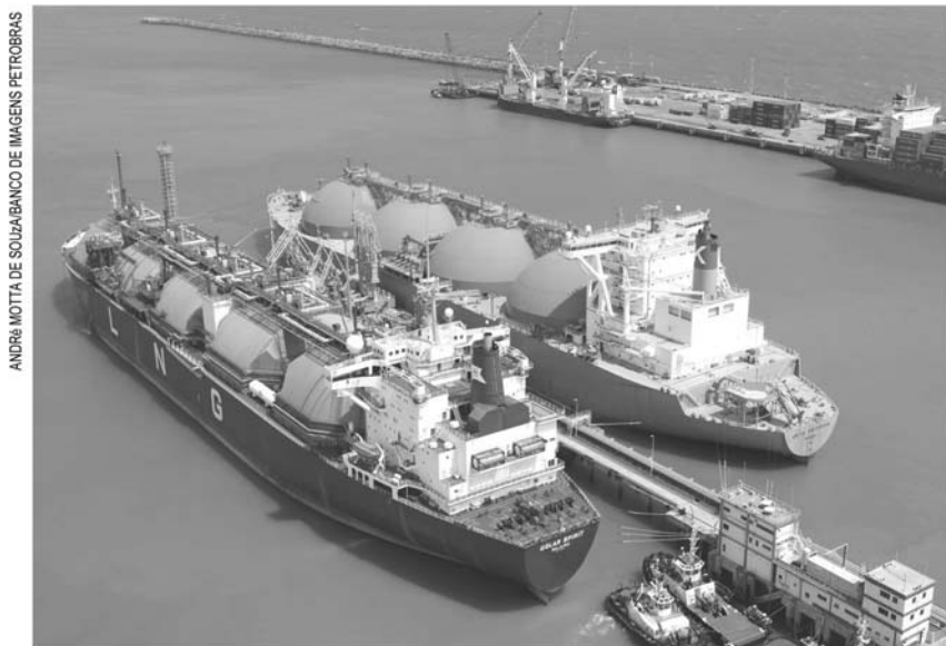
Figure 3.11 Terminal for transferring LNG. In addition to the safety requirements related to operation in the presence of hydrocarbons, specific safety requirements for cryogenics must be considered. LNG , Liquefied natural gas.
