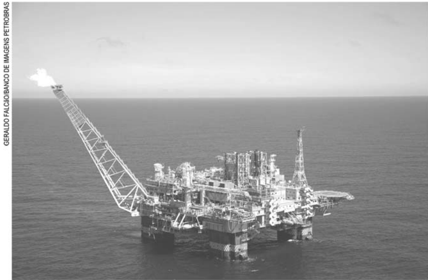
Figure 3.6 SS rig. SS, Semisubmersible.
