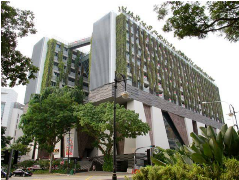
Figure 10.3. The Singapore School of the Arts building incorporates many of the traditional architectural responses to a hot and humid climate. The rectangular shape creates an envelope that is large compared to its volume (enhancing heat loss and exposing a small roof area to direct solar gain). The building is raised to access faster moving air, and the envelope is permeable to allow air to ventilate the building. (Source: School of the Arts, Singapore by Katmorro is licensed under creative commons)
