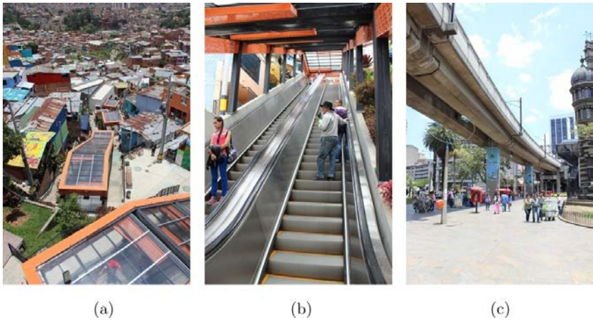
Figure 9.11. (a) Metro-cable in Medellín city, Colombia, (b) escalator system in San Javier Community and (c) detail of the escalator system. (Source: Photographs by Roberto Ghione)
