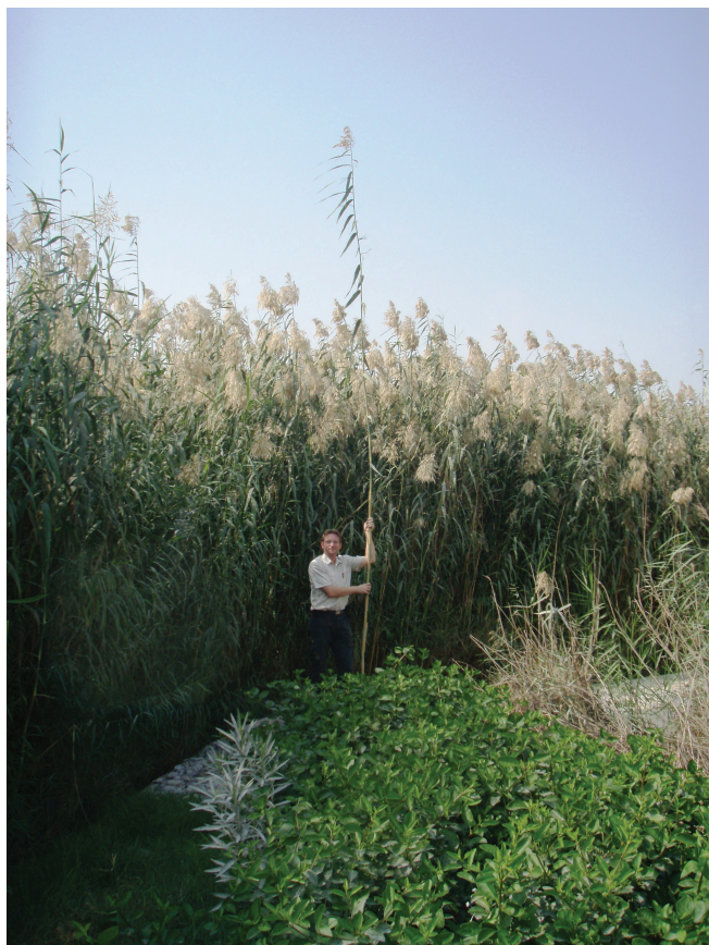
Fig. 13.2. A P. communis reed bed treating 25 to 30 m 3 of wastewater per day in Dubai. Photograph by W. Sievert, reproduced with permission from the Sustainable Sanitation Alliance (SuSanA) Secretariat under the Creative Commons License CC BY 2.0 ( https://creativecommons.org/licenses/by/2.0 ).
