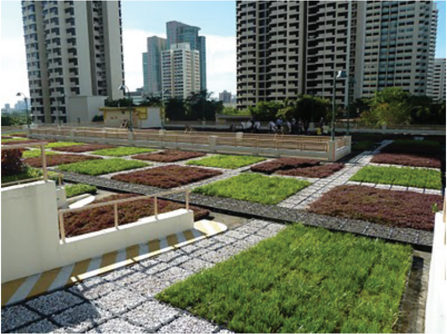
Fig. 3.2. Intensive roof on the top of a carpark
