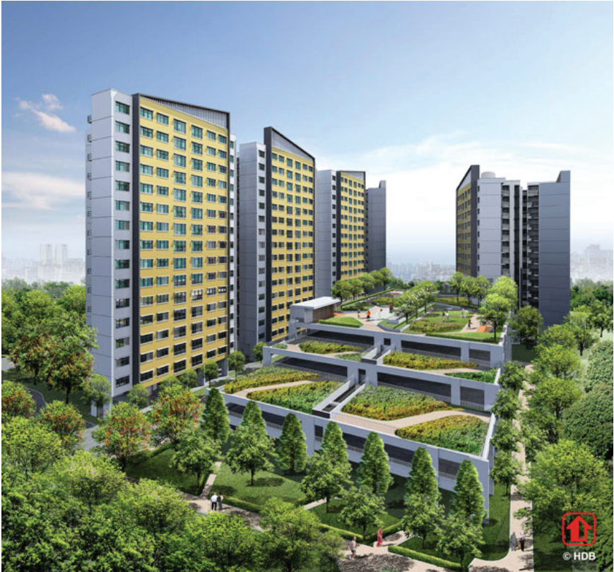
Fig. 3.6. Tampines Green Terrace, Singapore
